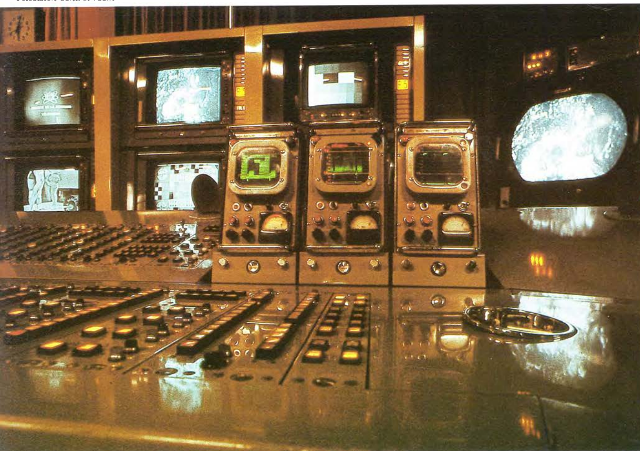
Television control room
