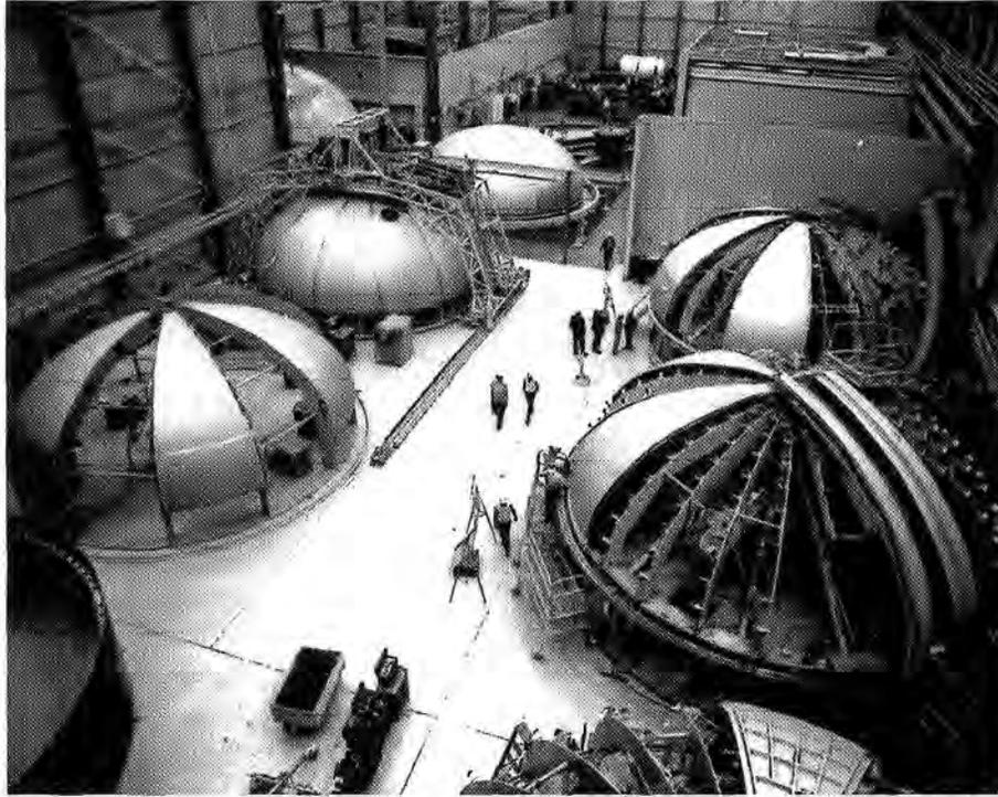
Gores being welded to bulkheads for the S-II stage of the Saturn V. (Source: Roger Bilstein, *Stages to Saturn* [Washington, DC: NASA SP-4206, 1980; reprint, Gainesville: University Press of Florida, 2003], p. 221)
